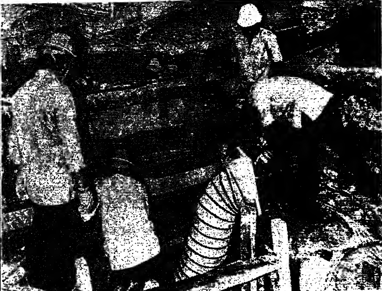
Rescue workers pumping air into a tunnel dug under the collapsed New World Hotel in Singapore to help possible survivors.
